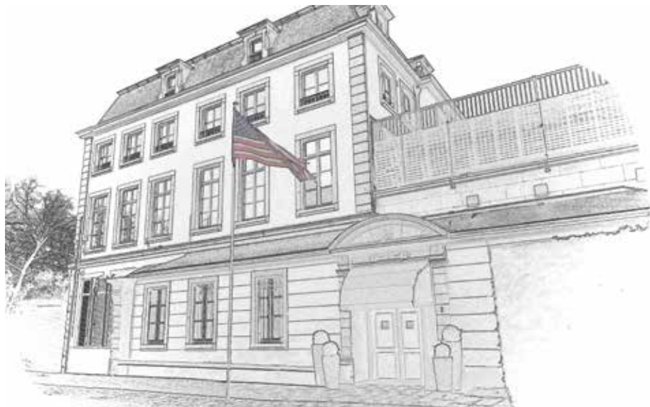
Whitlock Hall Brussels, Belgium
