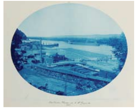
Old Pontoon Bridge at North McGregor Lane, 1885
