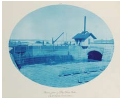
Inner Faces of Dry Dock Gates (Des Moines Rapids Canal), 1891
