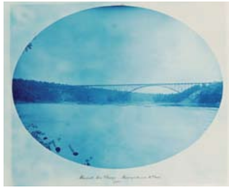
Marshall Avenue Bridge, Minneapolis and St. Paul, 1889
