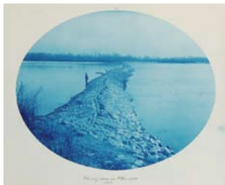
Closing Dam Otter Chute, 1889
