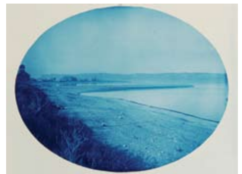
Breakwater at Lake City, Minnesota (Lake Pepin), 1889
