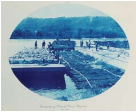
Construction of Rock and Brush Wingdam, 1891
